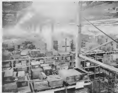
Storehouse section (3) of the big Austin building brings together under one roof a large portion of the refinery's material supplies; provides safe, neat storage for both bulky items and small parts.
